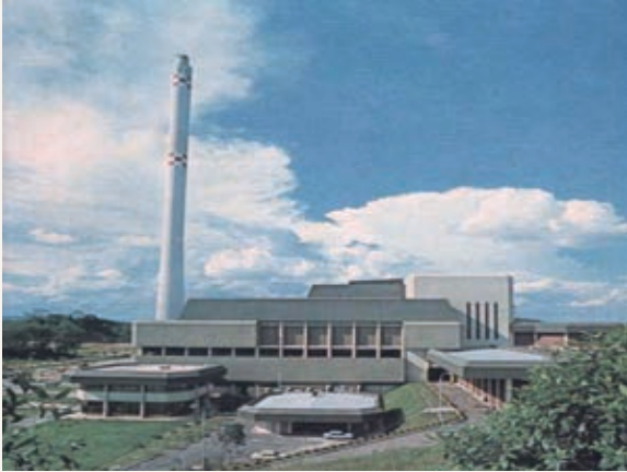
Ulu Pandan Refuse Incineration Plant
