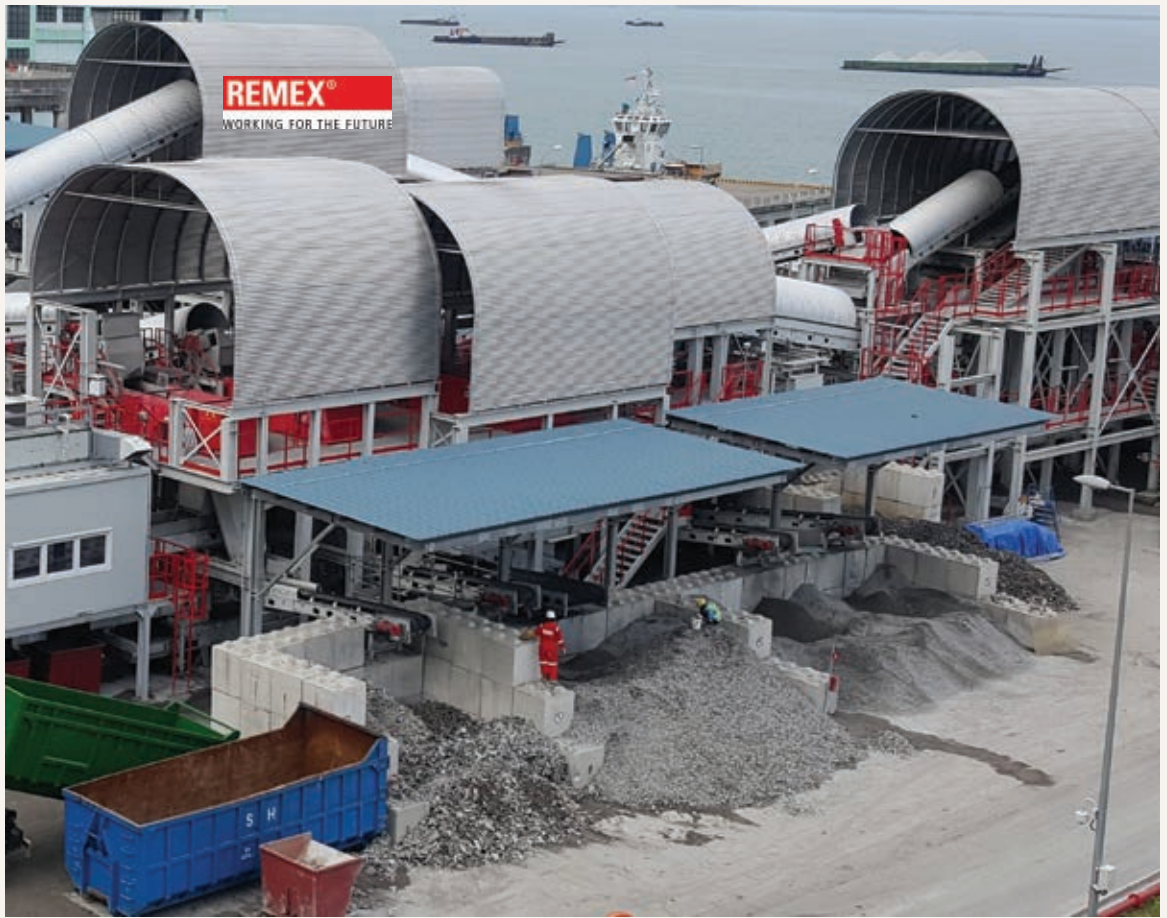
Incineration bottom ash (IBA) is processed at the REMEX metal recovery facility to recover ferrous and non-ferrous metals Photo: REMEX
